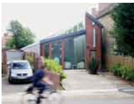
Top: A dilapidated, single-storey doctor's surgery previously occupied the site.
