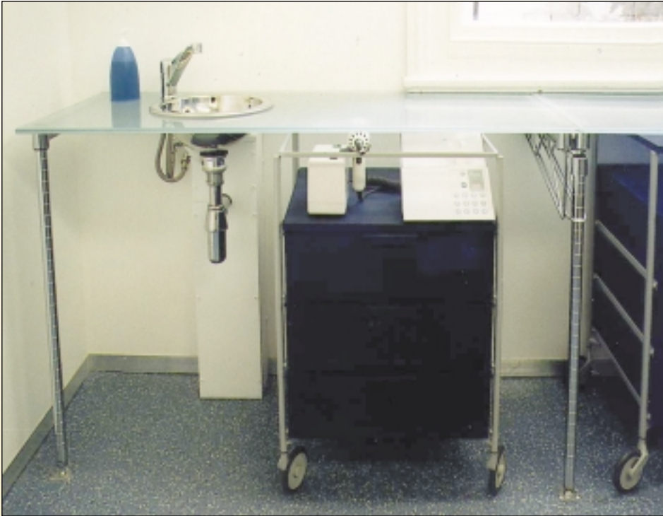
Figure 10: The support structure and the sink fittings
