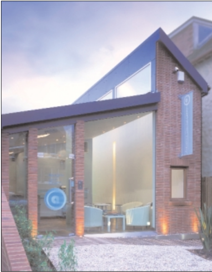
Figure 2: The outside of the new practice from the front
