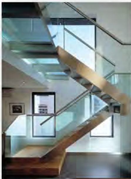
Each practice design incorporates an individual design feature, such as this elegant floating stainless steel and glass staircase (Pentangle, Newbury)
