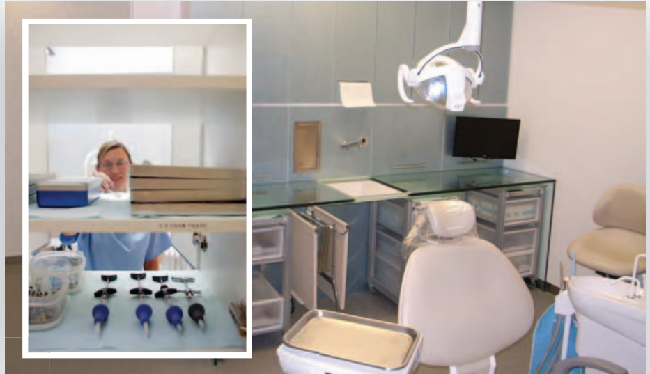
Double-sided Steri-Walls are accessible from both the surgery and the staff area behind, so bagged and sterilised equipment can then be loaded directly from the latter ready for use in the surgery to be unwrapped in the presence of the patient (Advance Dental, Chelmsford)
